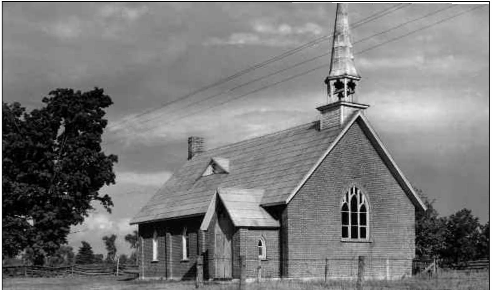
The original church on this site was consecrated in 1878 but later burned to the ground. This red brick church replaced it in the early 1900s.
